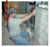
Too often, accidental contact from an electrical worker closes a circuit and produces an explosive arc flash.
